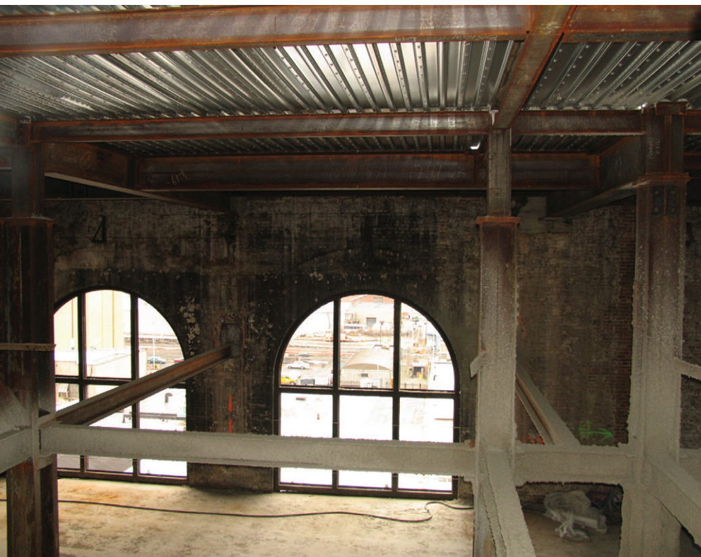
Additional steel framing facilitated the development of individual condominium units inside the old power generation station. Photo: Wexler Associates.
