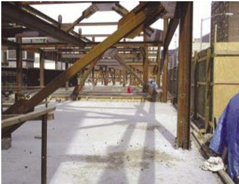
Lateral force resistance is provided by braced frames. Brace members were typically HSS shapes.
